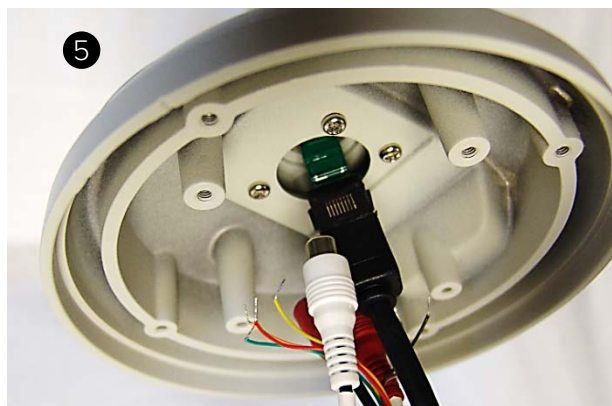
5. Connect all cables and verify camera is operating properly.
