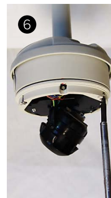
6. Attach the camera to the ceiling mount and secure the cover dome properly.
