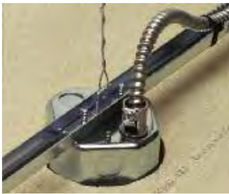
6 Install cable with connector (not included).
