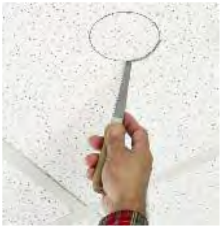
2 Cut a 4-1/16" diameter hole in the ceiling tile.
