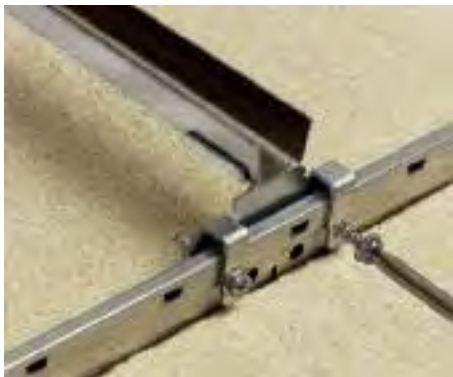
5 Option Use sheet metal screws – where required by local code – to hold ends securely on grid (screws not included).
