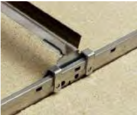
4 Position ends of support bar over the ceiling grid (tees).
